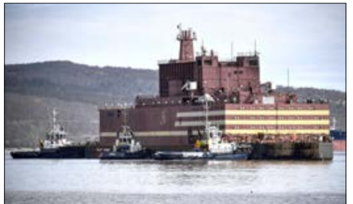
■ Floating power unit Akademik Lomonosov being towed to Atomflot moorage of the Russian northern port city of Murmansk
